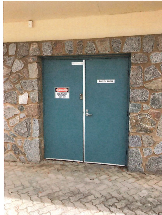
ENTRY TO SWITCH ROOM
